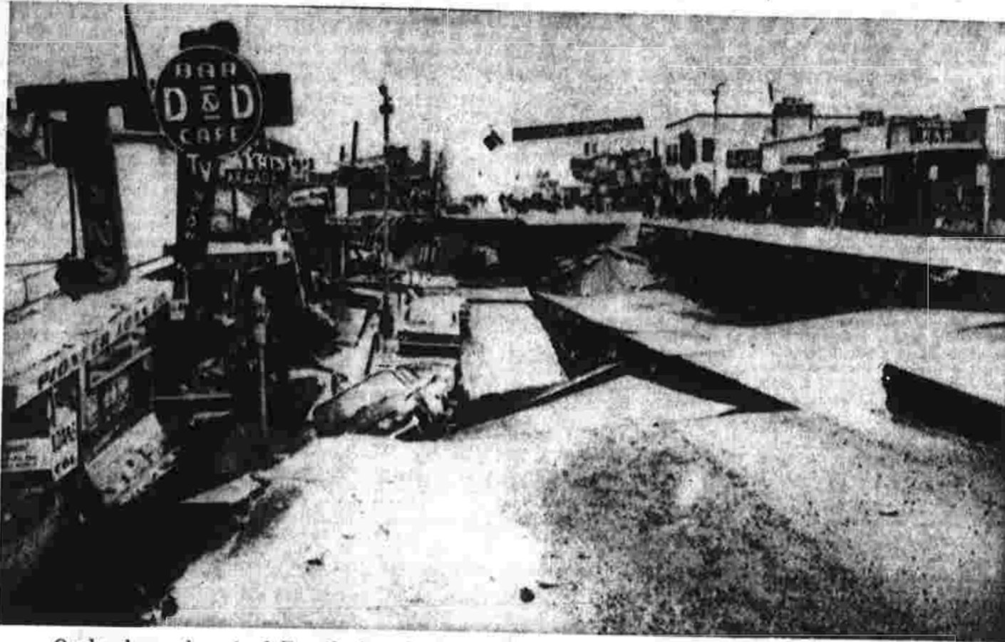
Quake dropped part of Fourth Ave. in Anchorage ten feet below former level. (AP Photofax.)
